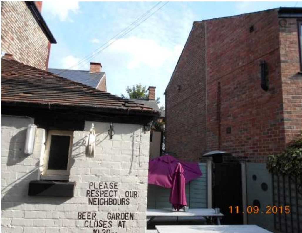
Rear Of Trevor Arms and gable wall of No. 19 Stanley Grove
